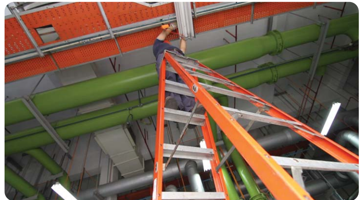
Test points can be far apart, or high above the ground.
